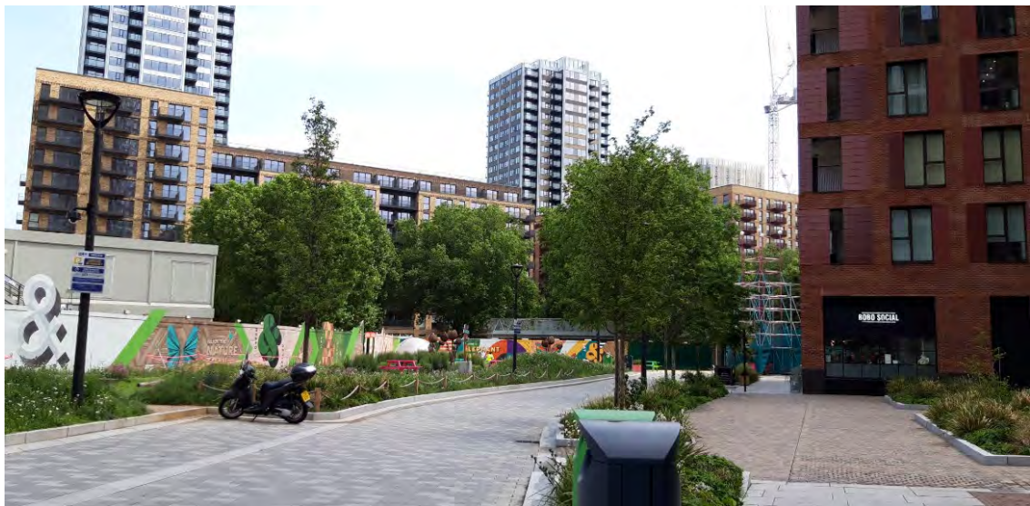
Part of the site's southern frontage, looking along Deacon Street, with Plot H2 on the right hand side, Plot H4 and H5 in the distance.
